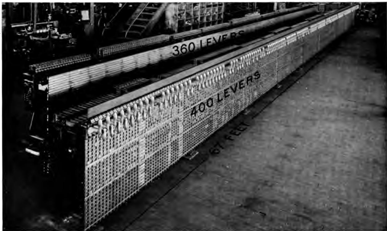
G. R. S. Electric Interlocking Machines, Grand Central Terminal, New York City
